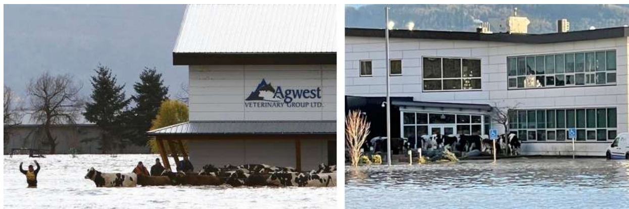
Figure 2. Pictures of the Agwest Veterinary barn and clinic during the 2021 BC Flood.
